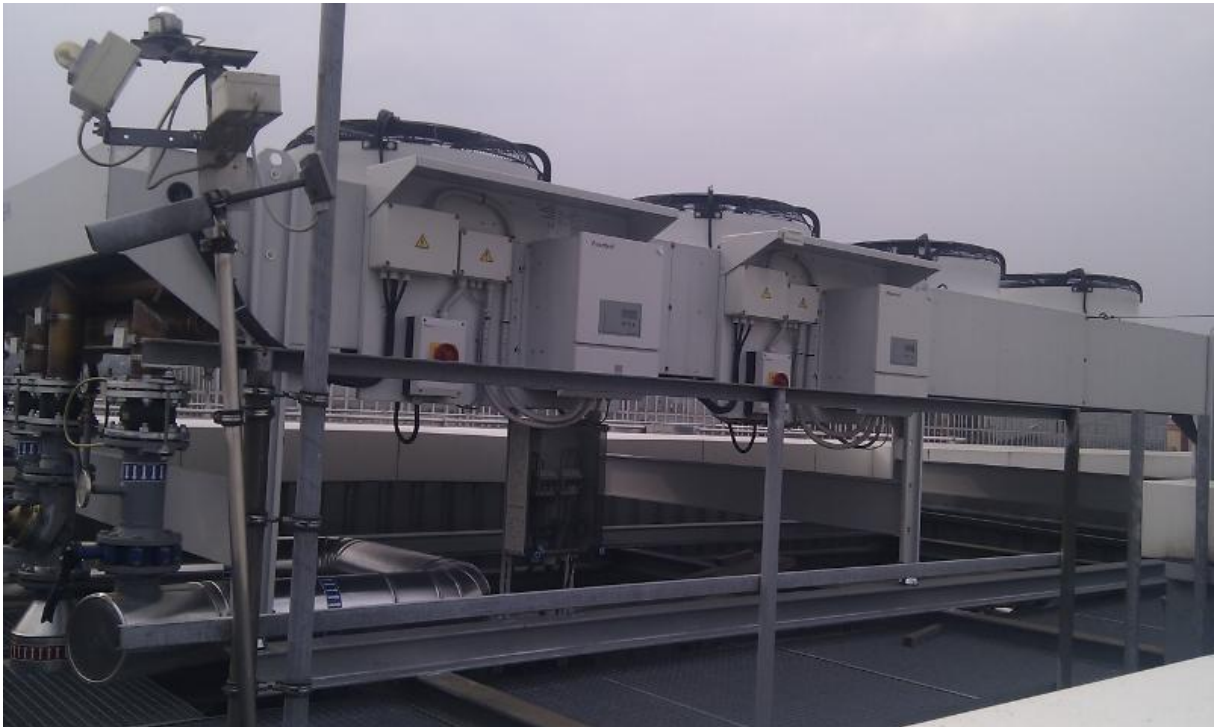
Fig A2.4: Roof cooler (Brandl 2012)
