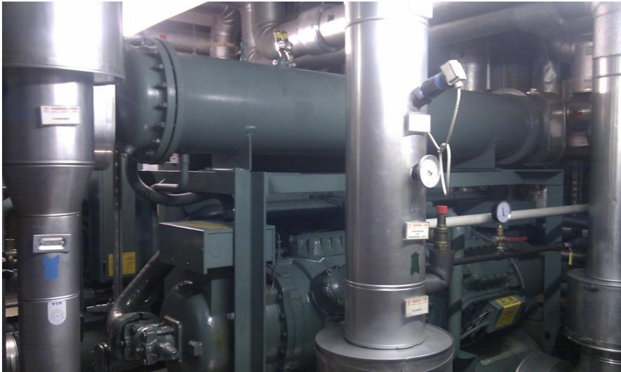
Fig A2.2: Cooling machine (Brandl 2012)
