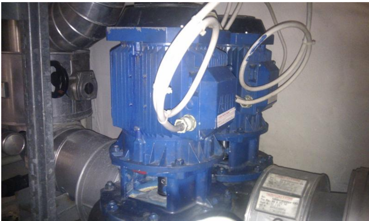
Fig A2.3: Cooling water "twin" pump with 6kW power (Brandl 2012)
